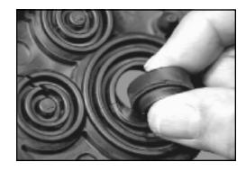
4.04 For existing cable, slit end seal from outside edge.
