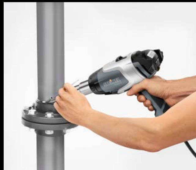
Welding plastic in tank and apparatus construction.
