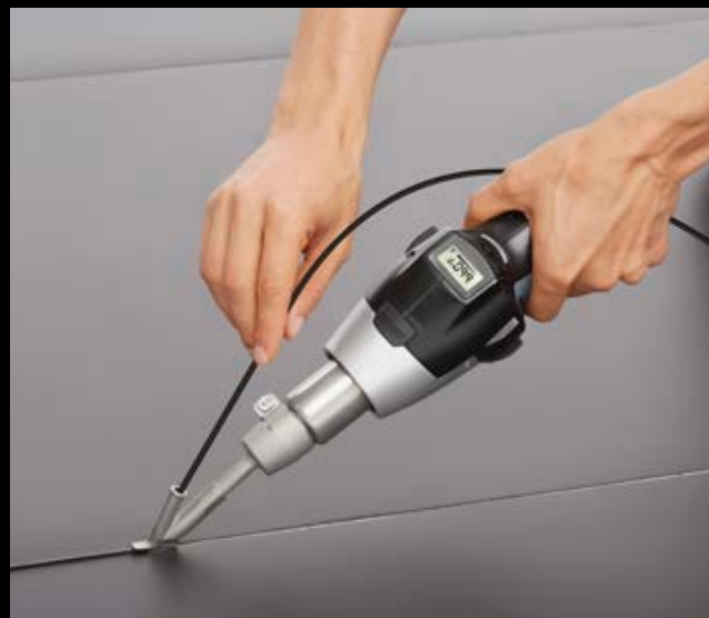
Welding linoleum floors.
