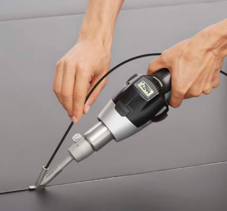
▲ Welding linoleum HG 2620 E
