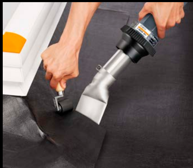
Overlap welding on a light dome.
