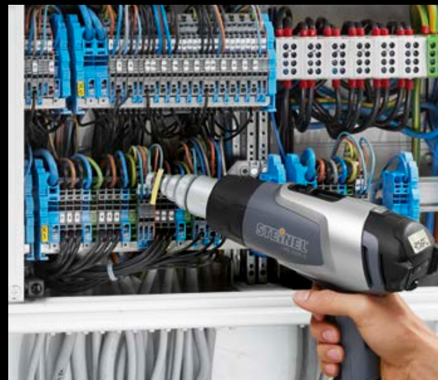
Shrinking cable sleeves in distribution cabinet
