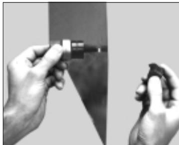
**2** Place 1/2" conduit die on 3/8" draw stud. Insert draw stud through pilot hole.
